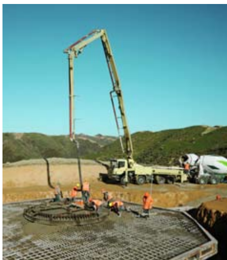
Top and left: The wharf at Oteranga Bay, which now has the gantry cranes installed and commissioned ready for the first deliveries expected in late October. Above right: A turbine foundation being poured.
