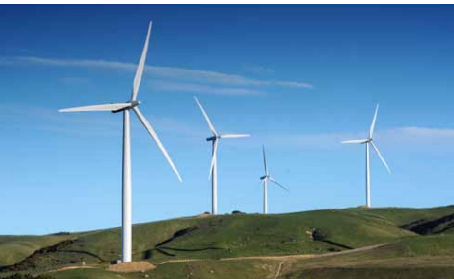
Turbines at Project West Wind generating clean, renewable energy.
