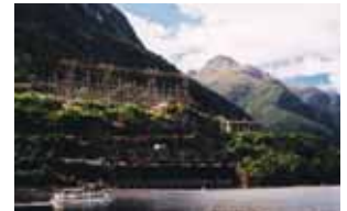
Lake Manapouri, looking towards the power station at West Arm.
