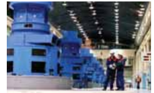
The Manapouri Power Station, which is undergoing major refurbishment.
