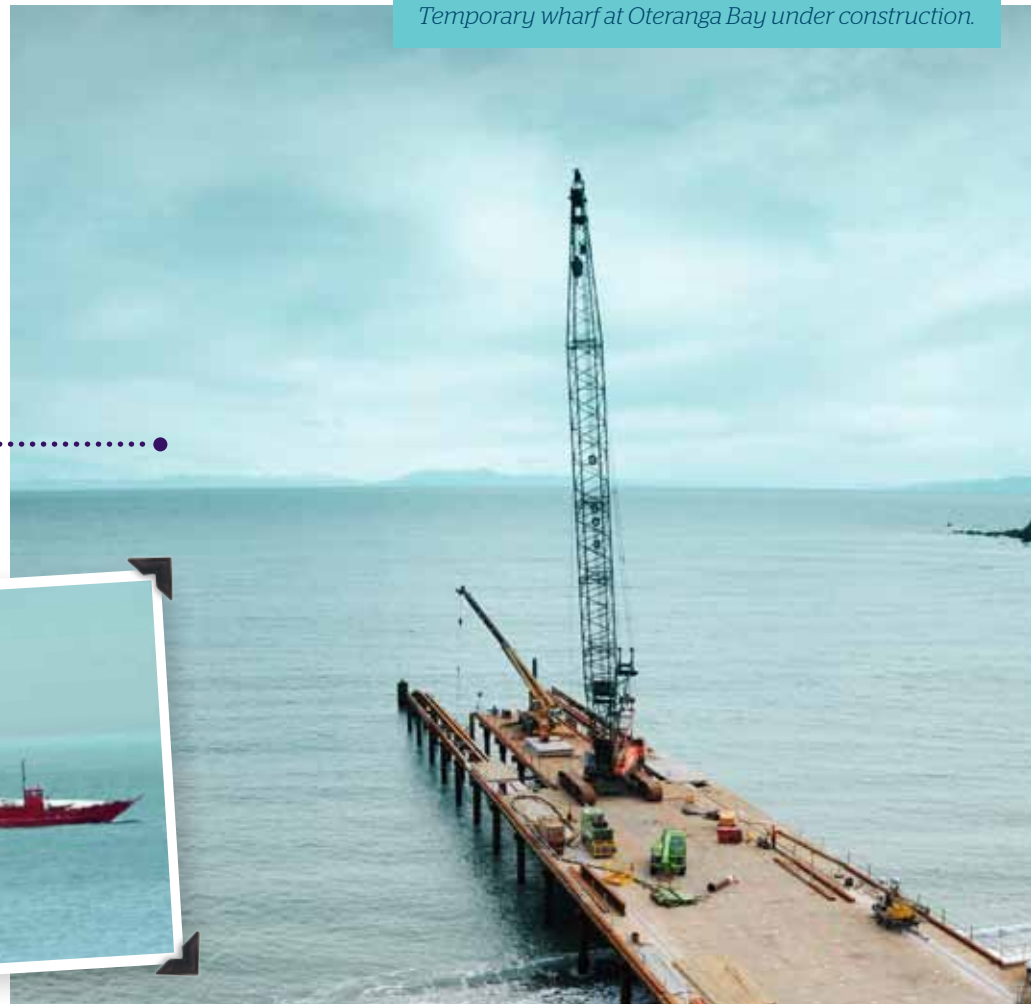
Temporary wharf at Oteranga Bay under construction.
