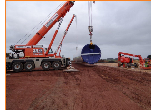
First tower section at Macarthur wind farm
