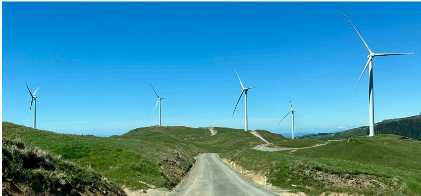
First five turbines in action.
