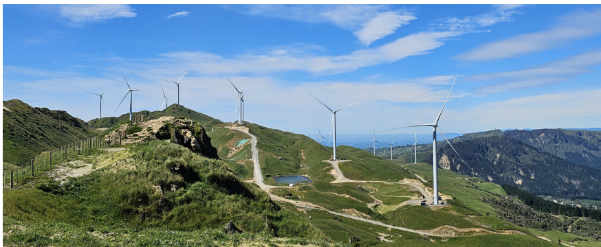
View of the Harapaki wind turbine site.
