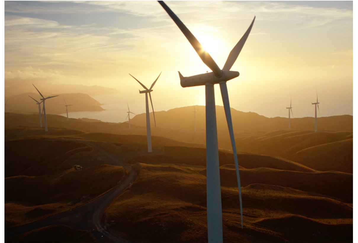
West Wind farm near Wellington
