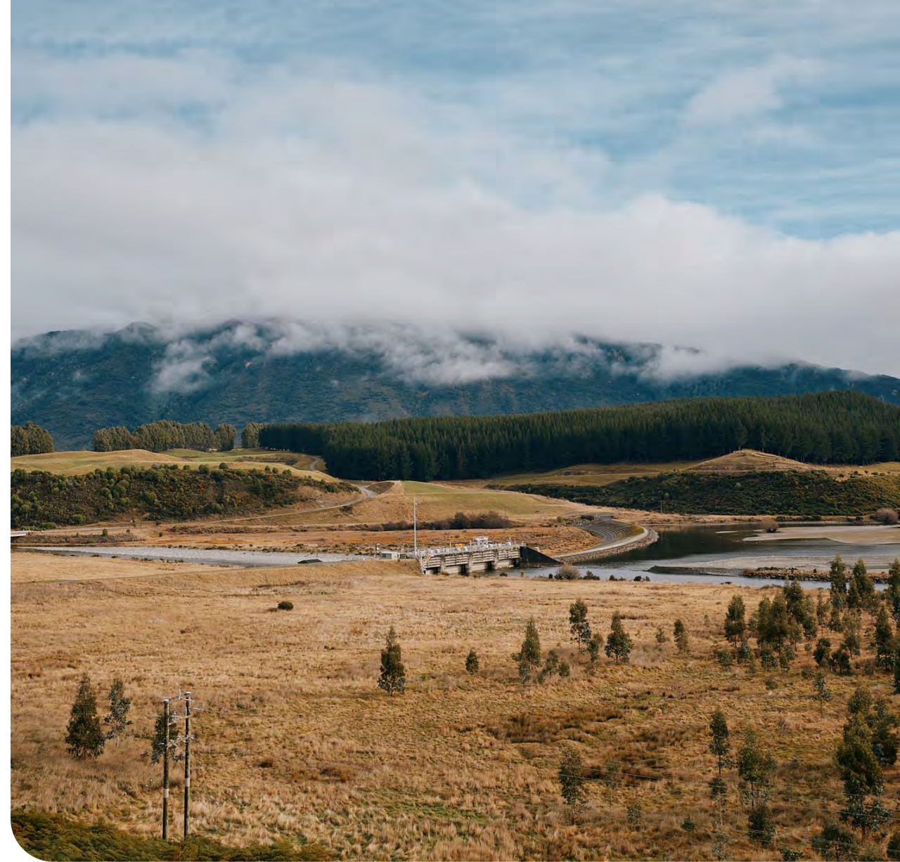
Manapōuri Lake Control structure
