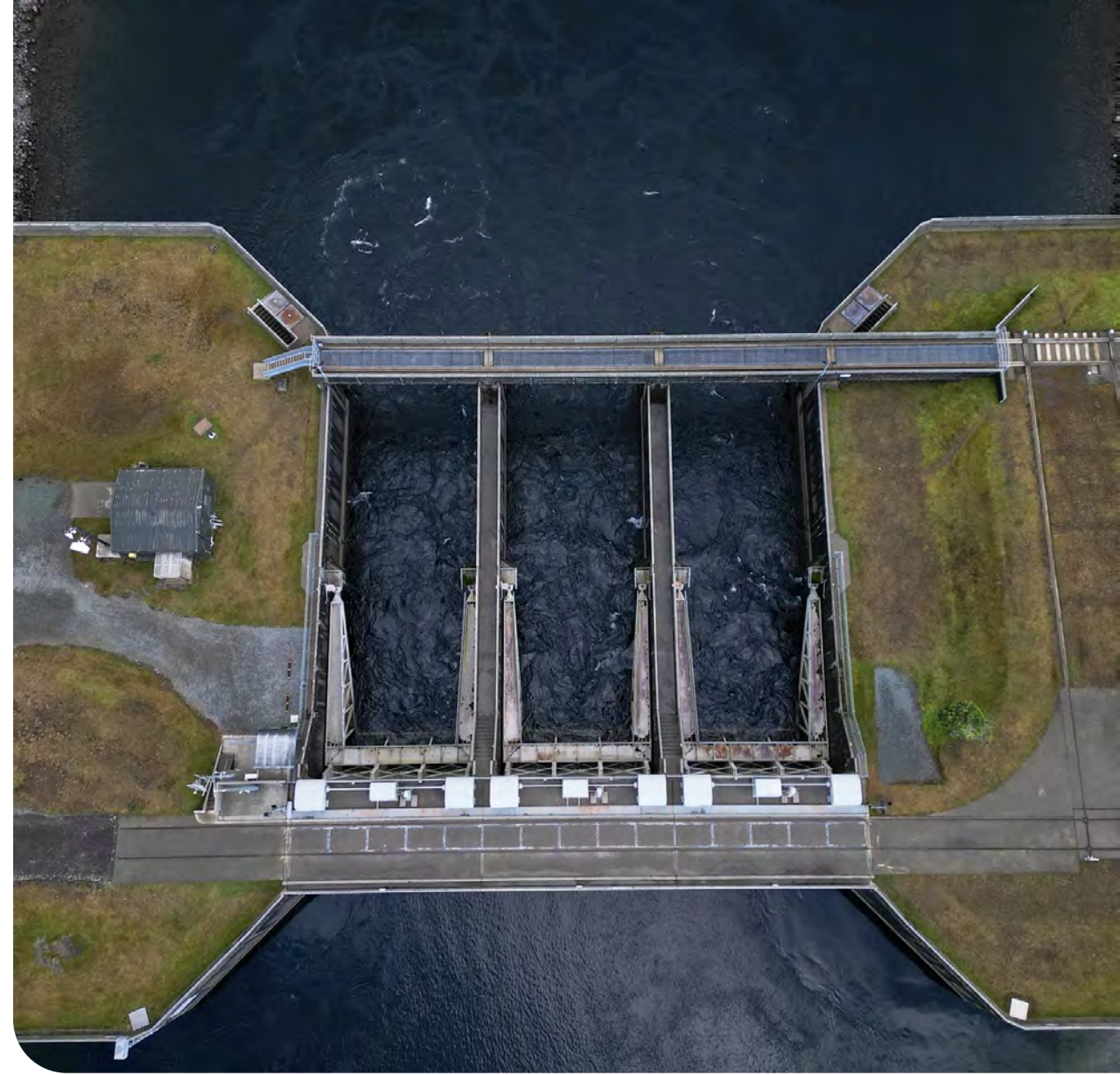
Te Anau Lake Control structure
