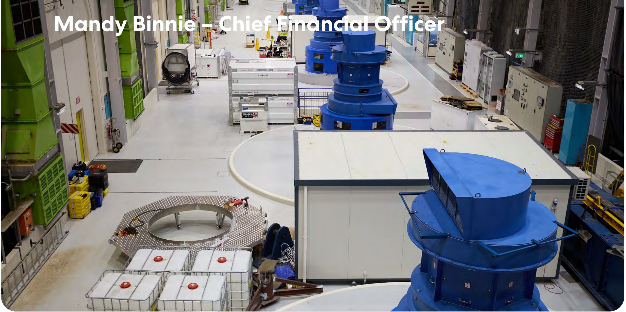
Meridian's Manapouri hydro power station
