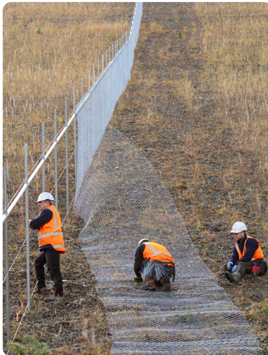
ABOVE: Fencing installation Benmore Power Station, Ōtematata.
