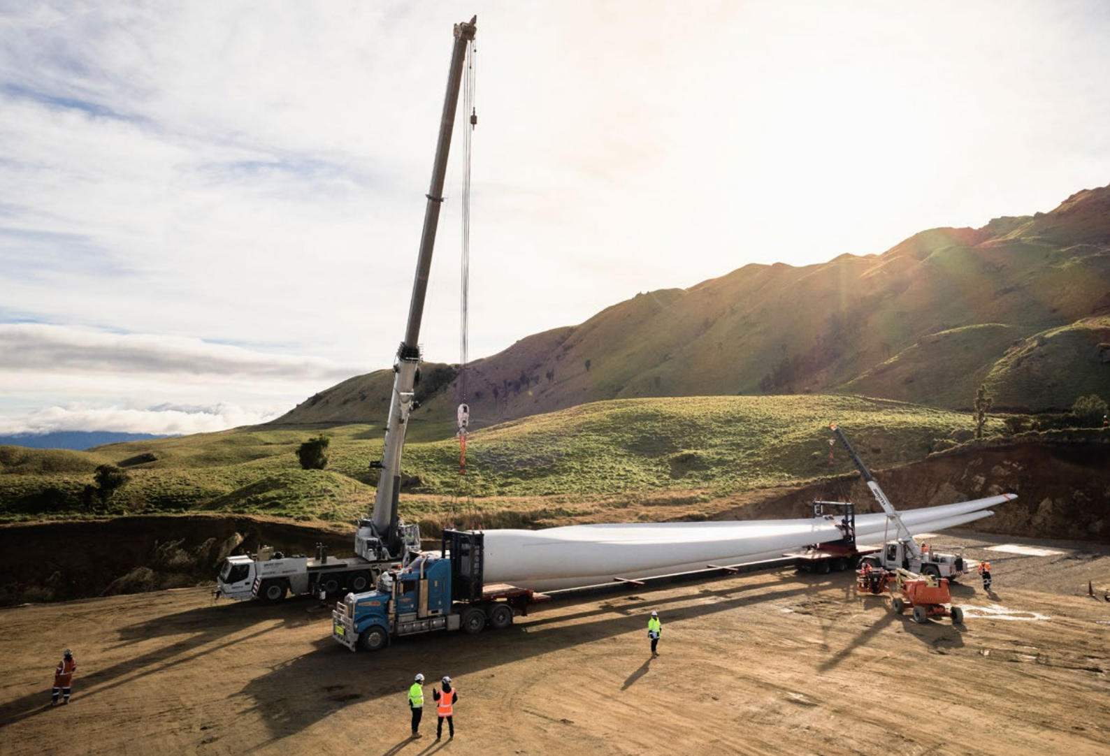
Harapaki wind farm construction, Hawke's Bay
