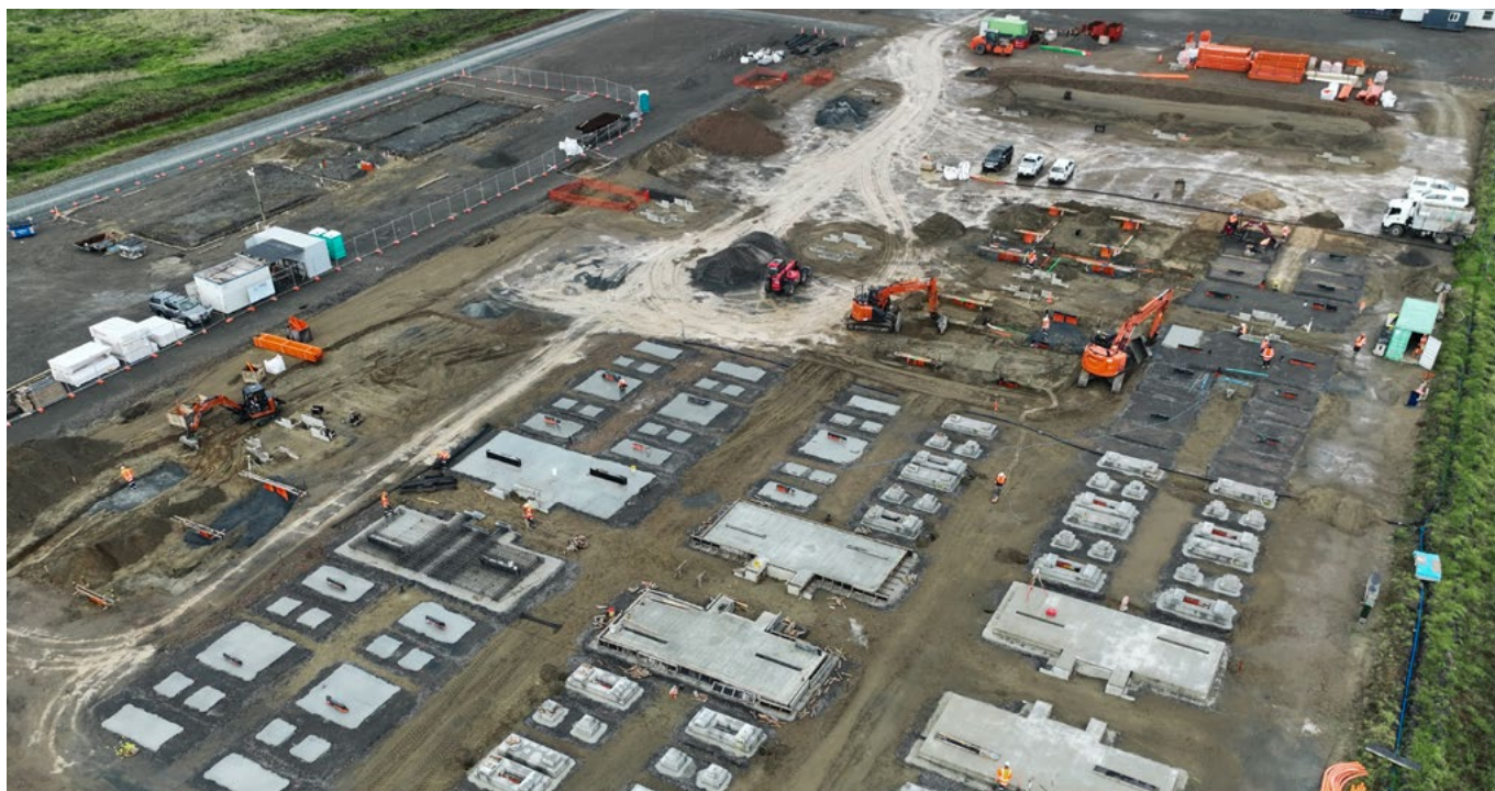
▼ Construction at the Ruakākā Battery Energy Storage System, near Whāngarei.
