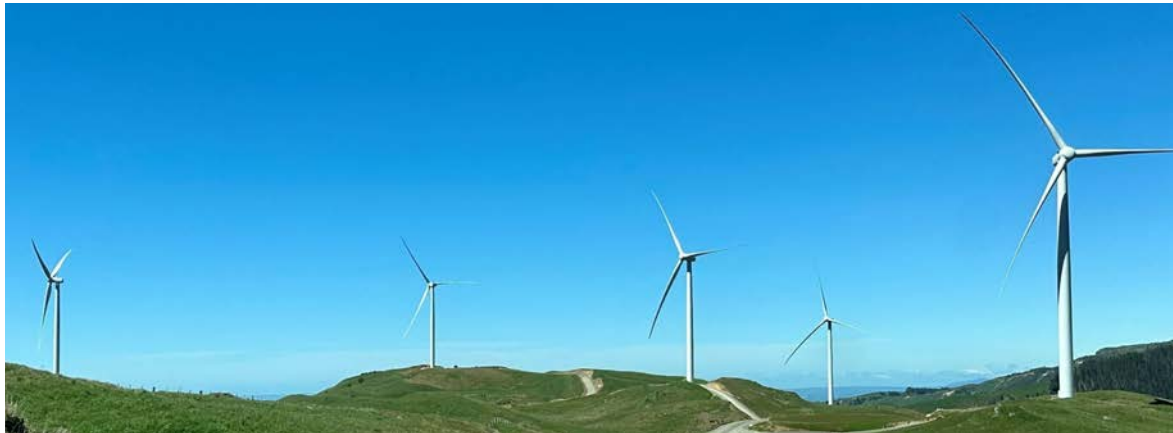
Completed string of turbines at the Harapaki wind farm in Hawkes Bay
