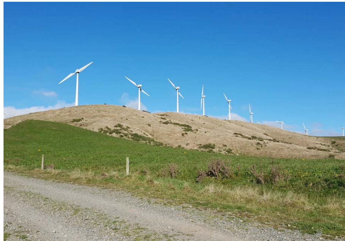
Existing turbines at the Te Rere Hau wind farm in the Tararua Ranges, outside of Palmerston North
