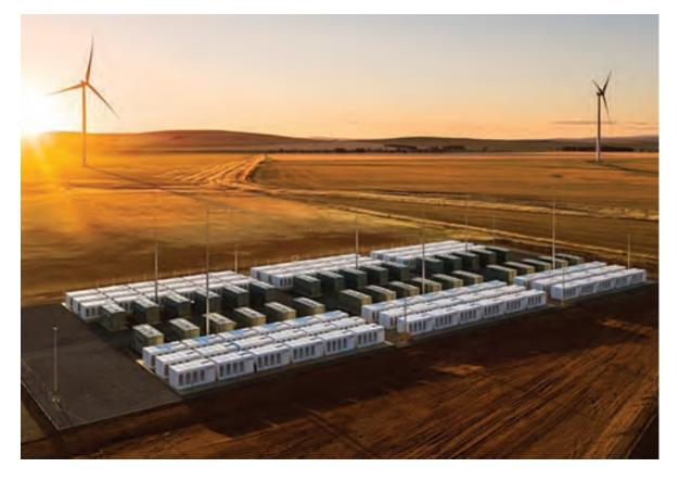
Tesla 100-MW/129-MWh energy storage system, Hornsdale Wind Farm in South Australia . Courtesy: Tesla
