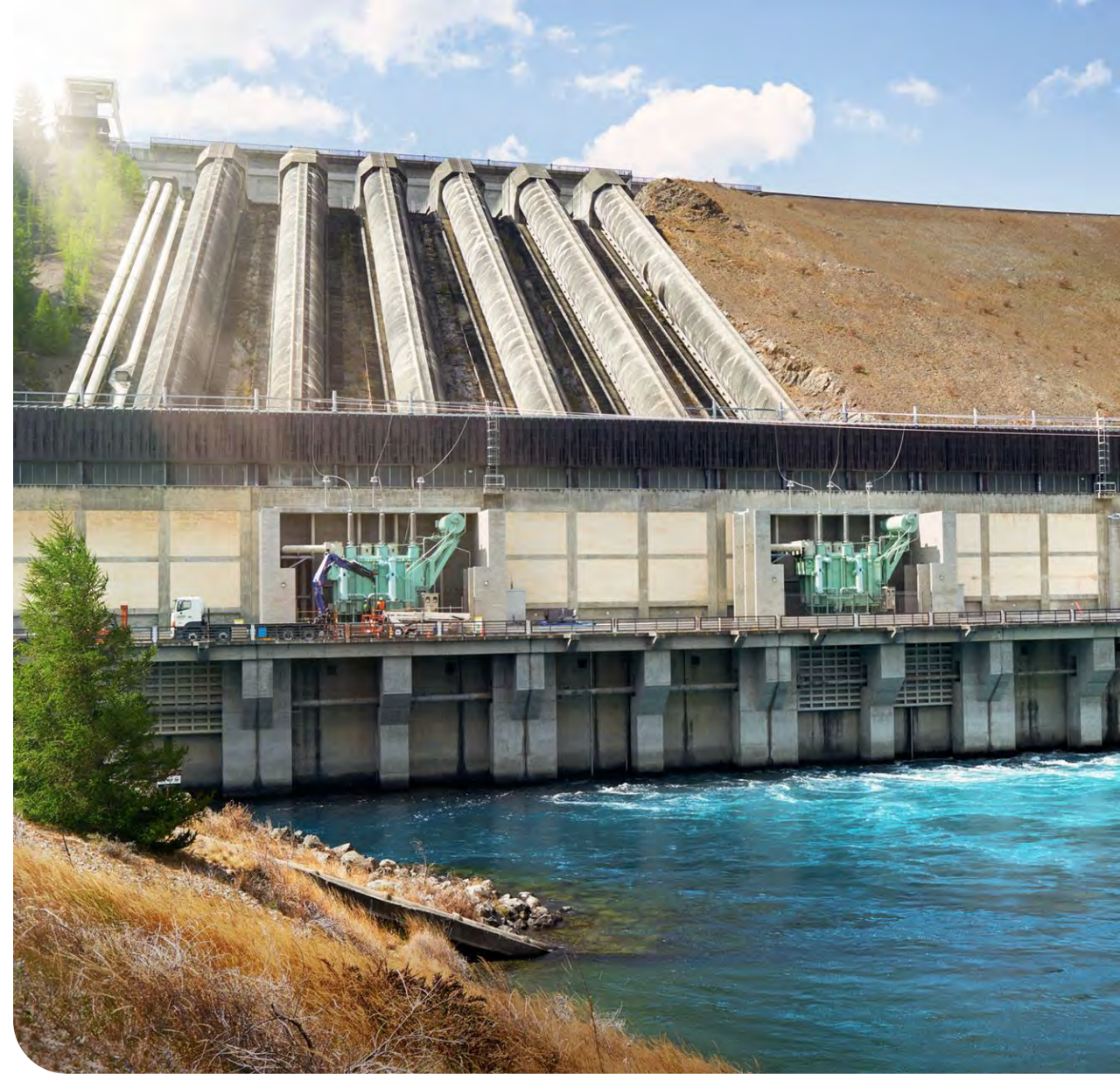
Benmore Power Station.
