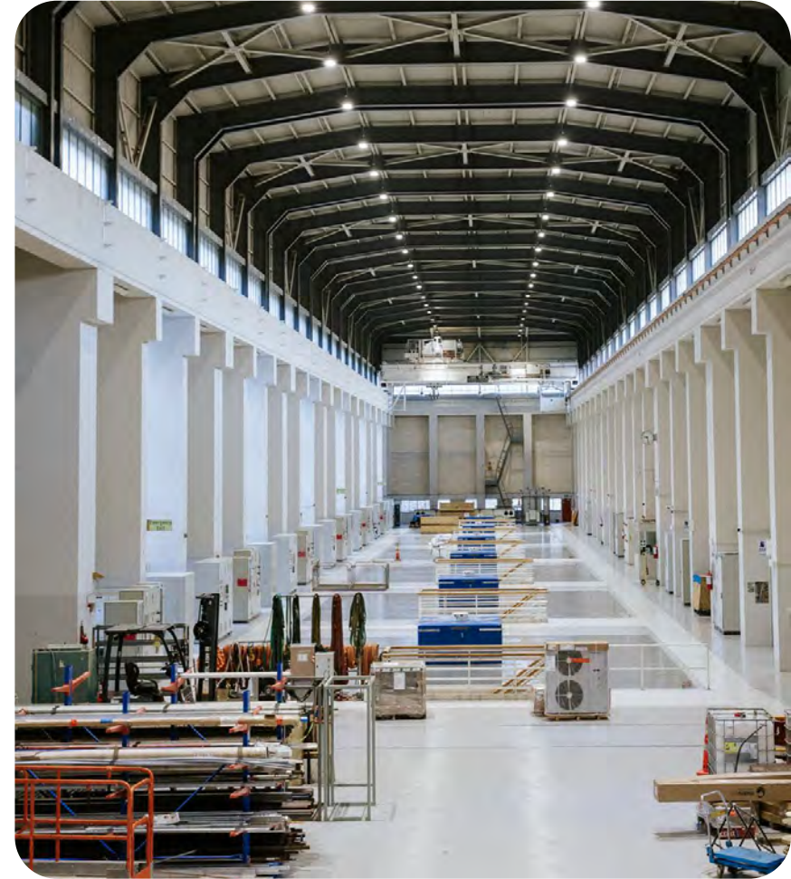
Benmore Power Station.
