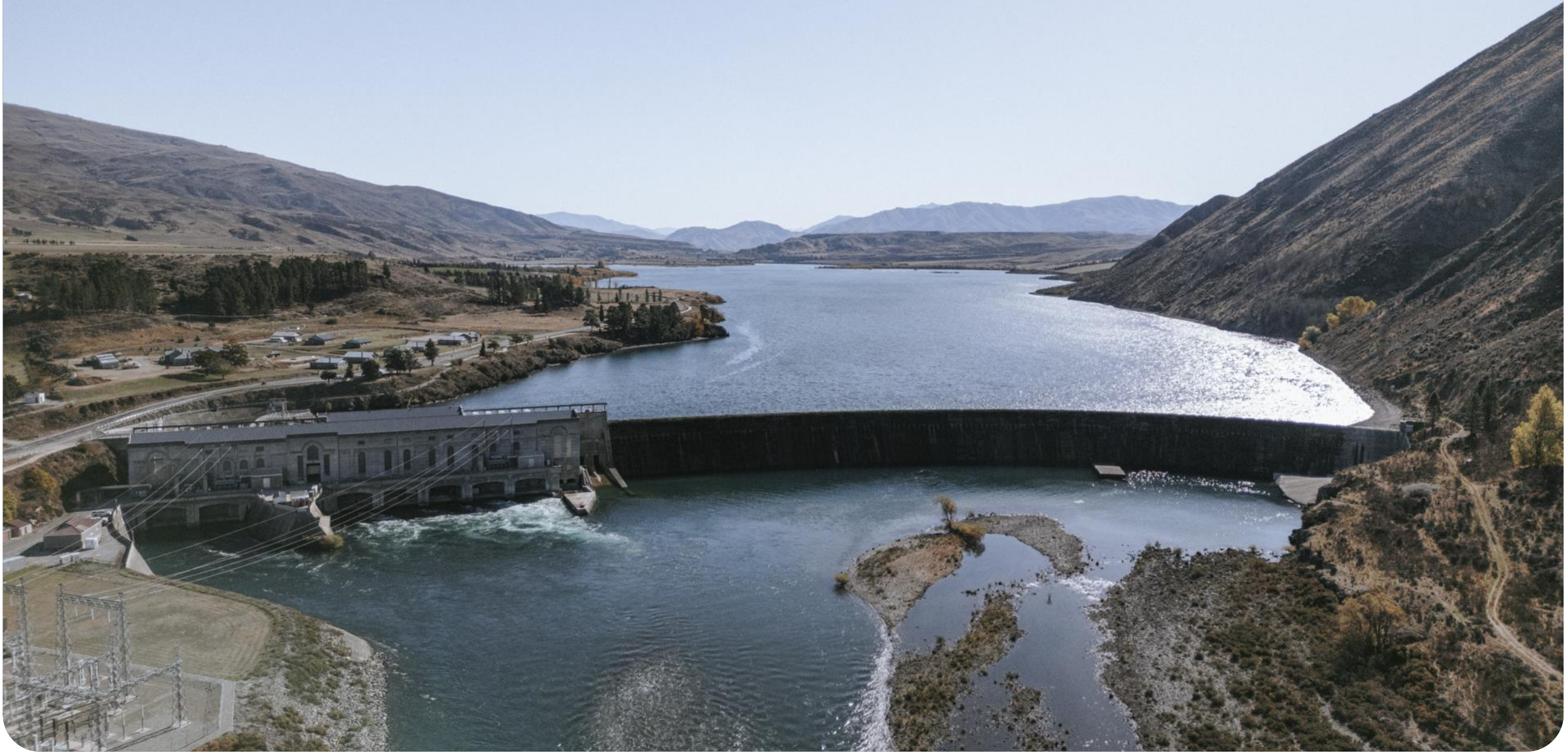
Construction of the Waitaki hydro power station originally began in the 1930's.
