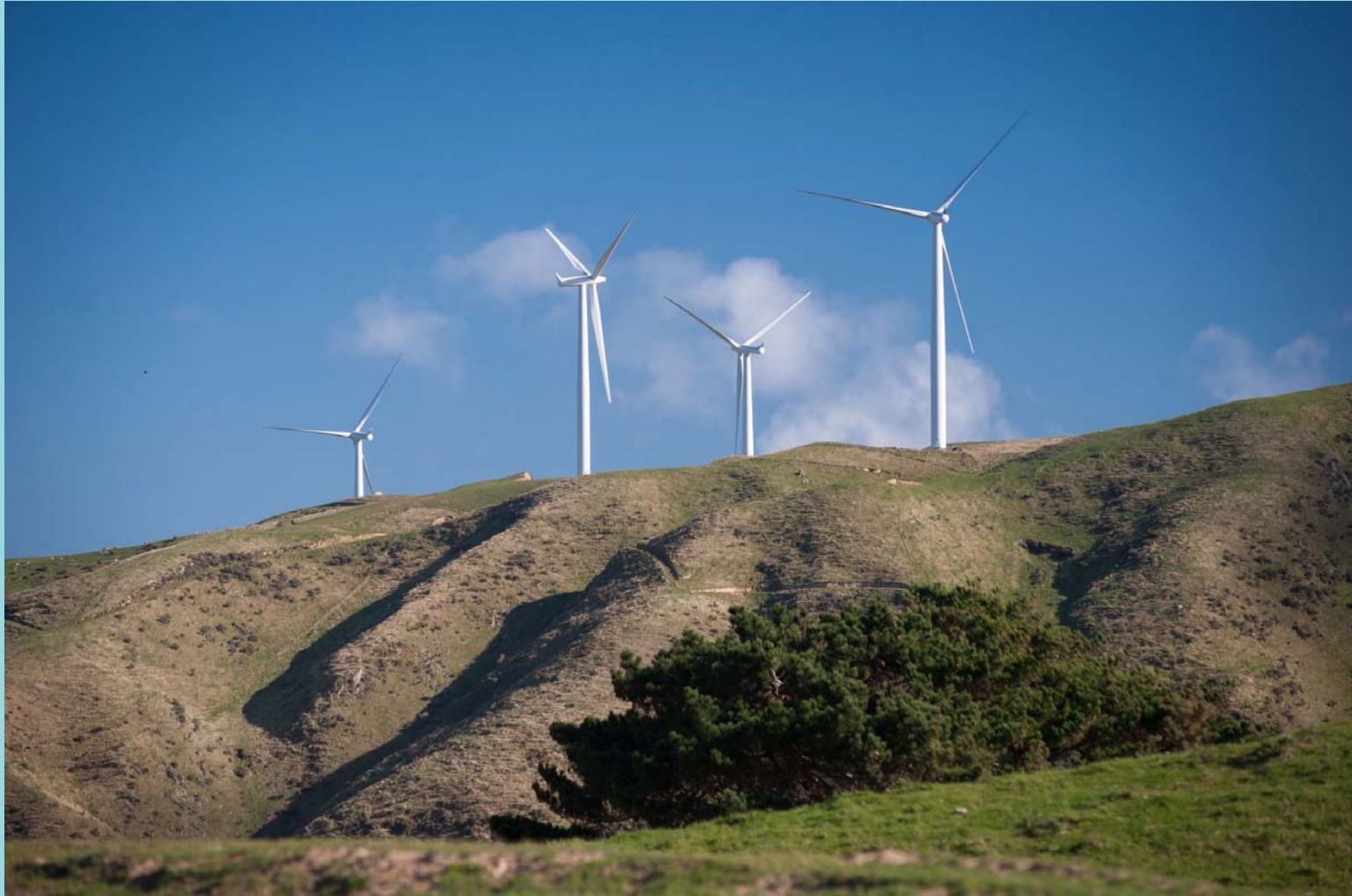
Mill Creek wind farm, Ohariu Valley, Wellington
