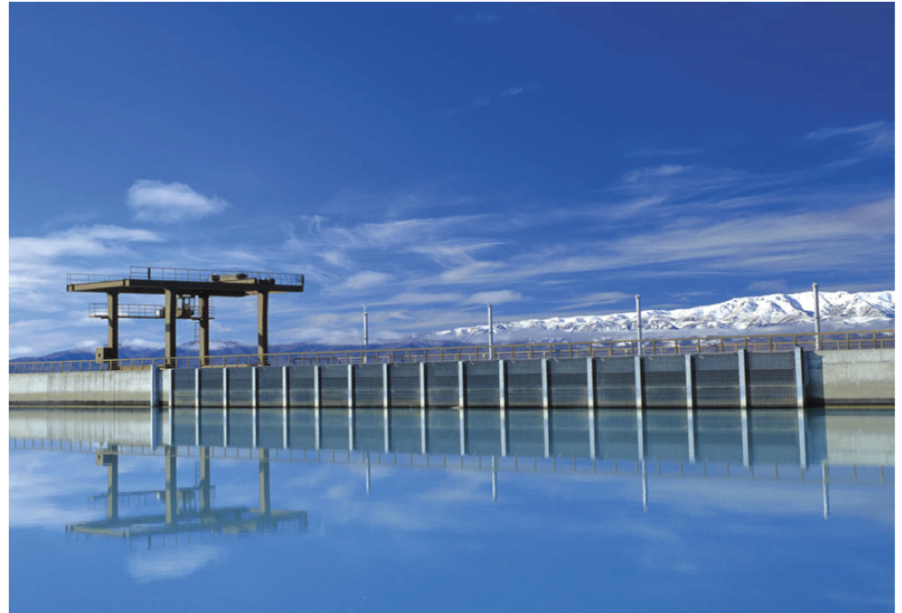
Control gates, Ōhau C power station, Mackenzie District
