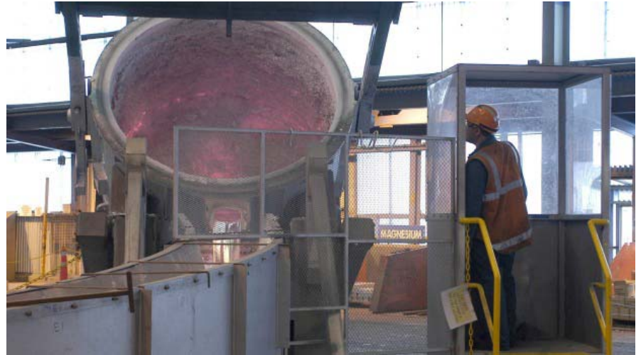
Tiwai Point aluminium smelter, Southland
