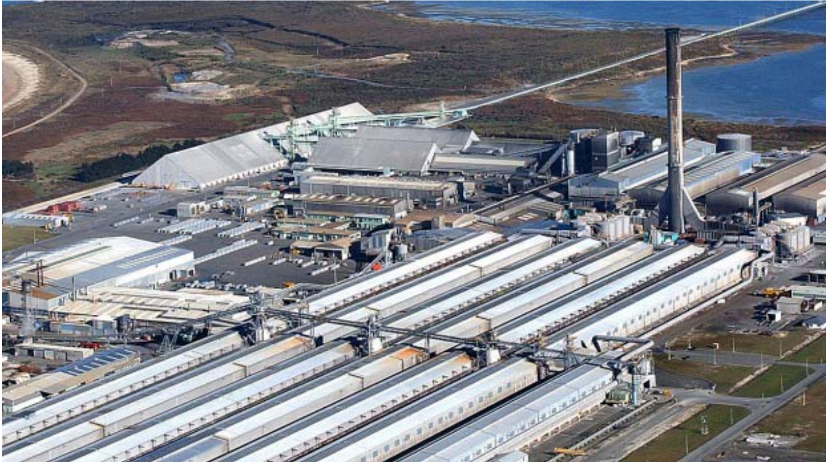
Tiwai Point aluminium smelter, Southland
