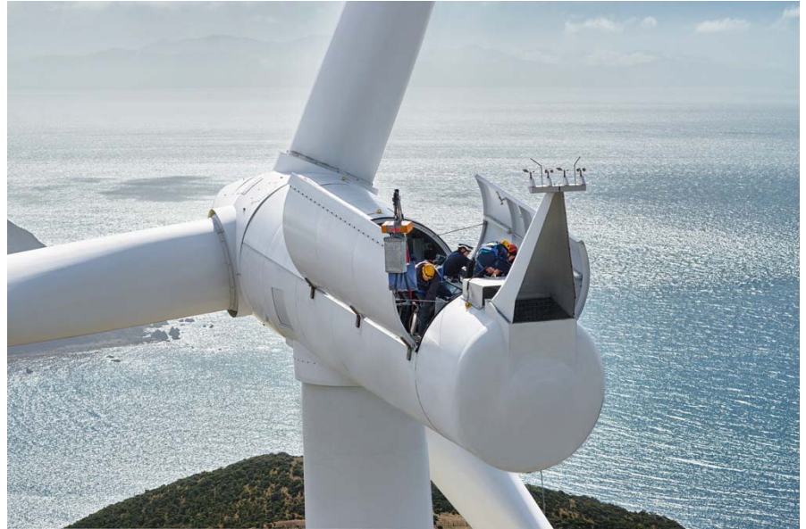
West Wind farm, Makara, Wellington
