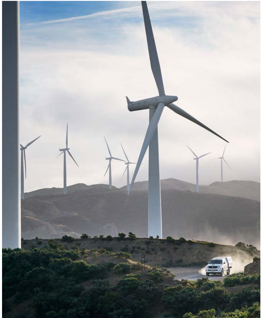
West Wind farm, Makara, Wellington
