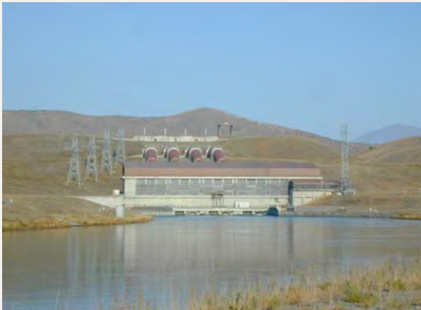
Image: Meridian's Ōhau B power station
