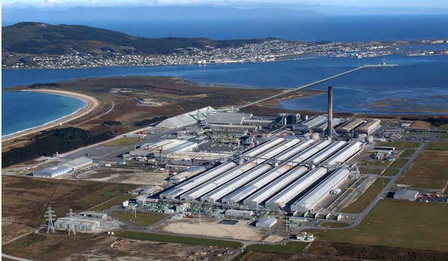
Image: NZAS smelter at Tiwai Point
