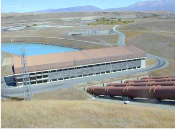
Image: Meridian's Ōhau A power station
