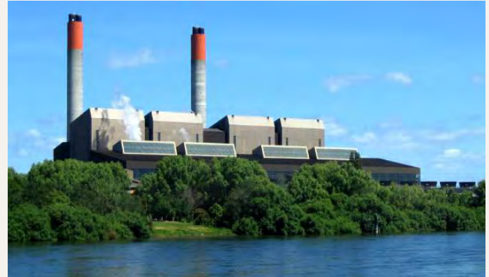
Image: Genesis Energy's Huntly Power Station
