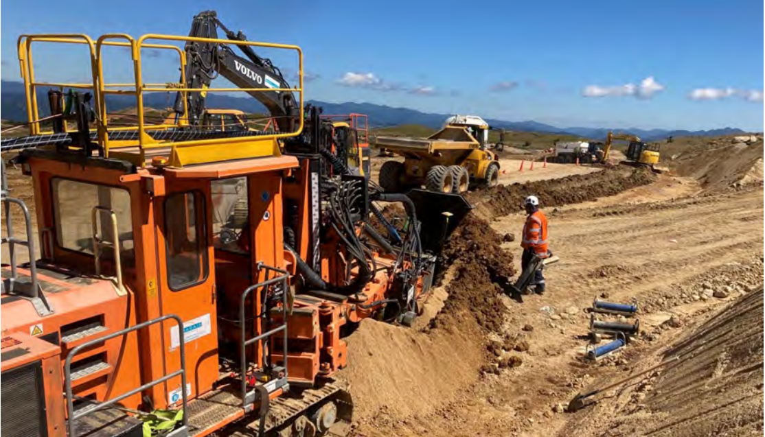
Cable trenching at Meridian's Harapaki wind farm
