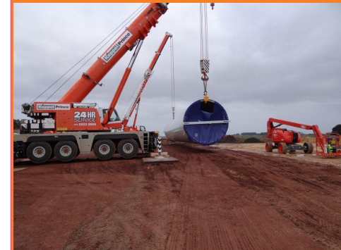
First tower section at Macarthur wind farm
