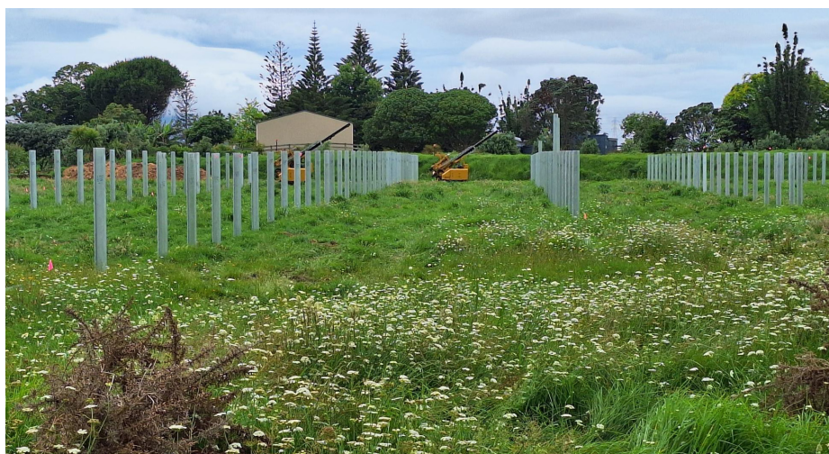
Metal piles that will be part of the supporting structure for the solar panels
