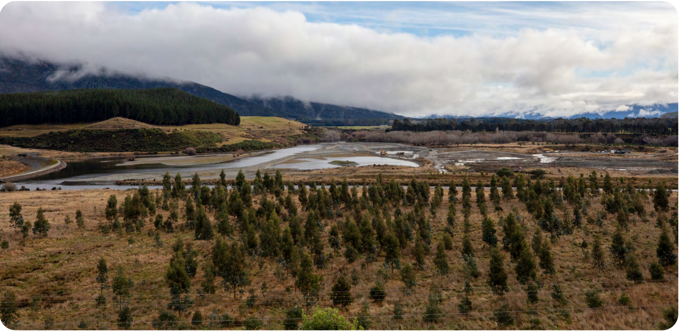
ABOVE: Waiau River above Mararoa weir, channel realignment project.
